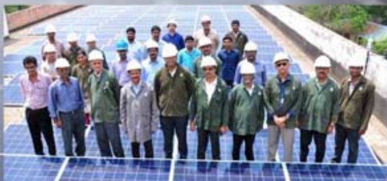
60 kWp Grid Tie Project at BPCL Cochin Refinery
